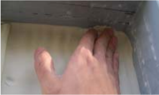
Figure 25 : Press the kaolin against the walls
