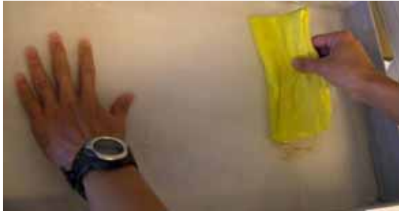
Figure 26: Disperse bubbles under the cloth
